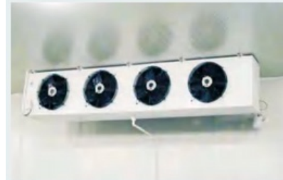
Air Cooler Installation Picture
