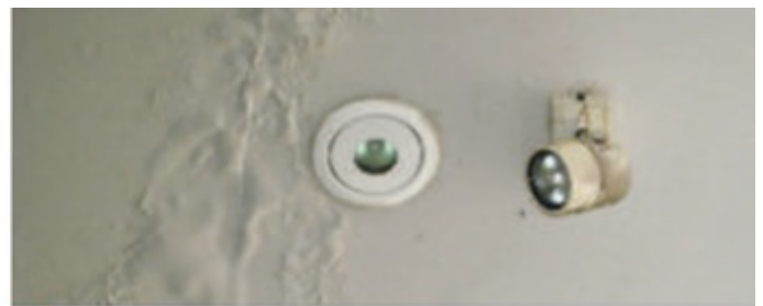
❌ Example: Gypsum Board Not humidity resistant
